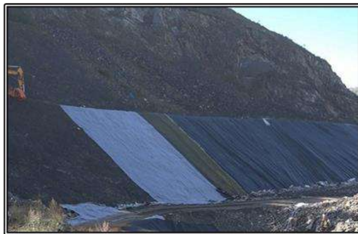
Figure 1 Setting up the geogrid
