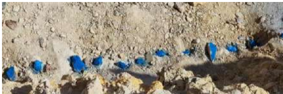
Figure 7 The row of drilled boreholes marked with blue spray [7]
