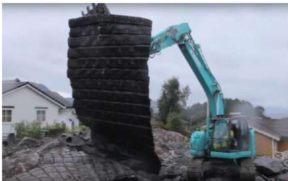
Figure 2 Placement of blasting mats on the blast field during blasting in urban areas [13]
