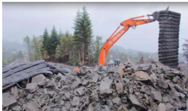
Figure 3 Removal of blasting mats after blasting from a muck pile with a hydraulic excavator [13]
