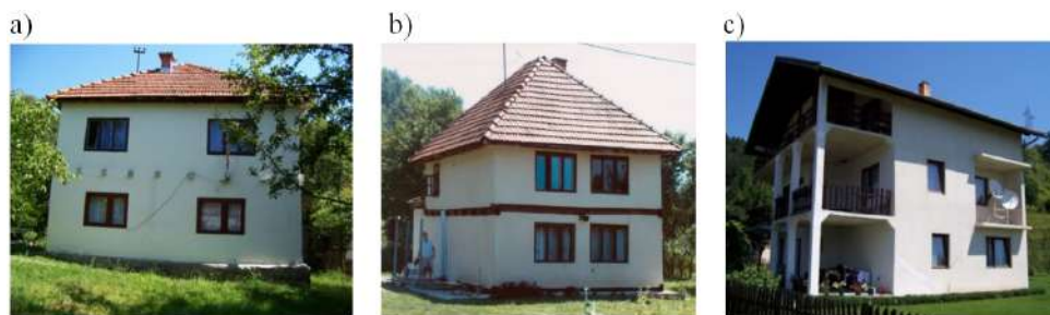
Figure 3. Residential buildings: a) with wooden construction between floors; b) built in timbered system; c) with derived AB horizontal and vertical cerclages
