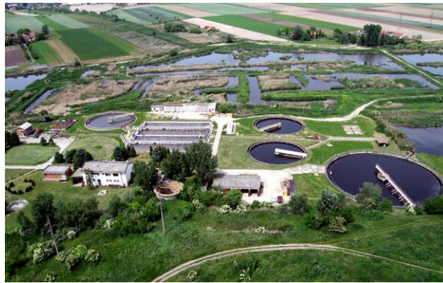
Figure 2. Waste Water Treatment in Subotica
