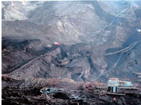
Fig. 5. Landslide on open-pit mine Kosovo-Belačevac
